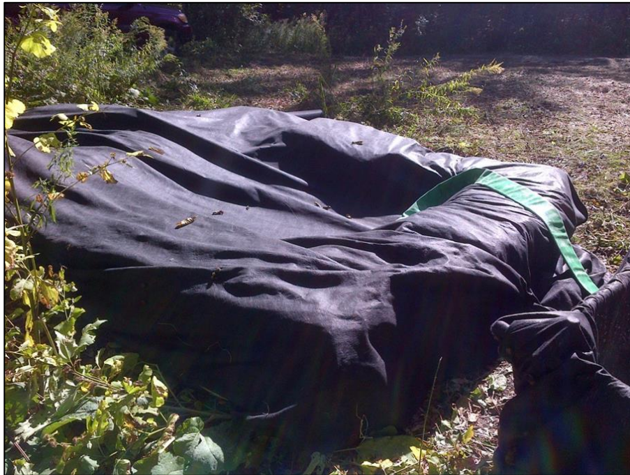
Diagram 2.12: Typical Dirty Water Treatment System (Hay Bales and Geotextile Fabric)
