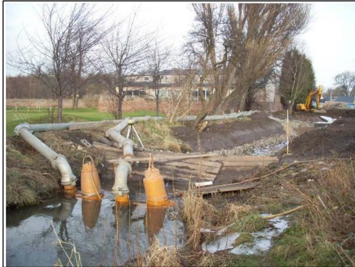
Diagram 2.9: Typical Arrangement for Full Isolation Over-pumping
