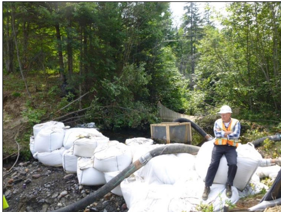
Diagram 2.14: Typical Cofferdam System (Industrial Sandbags)
