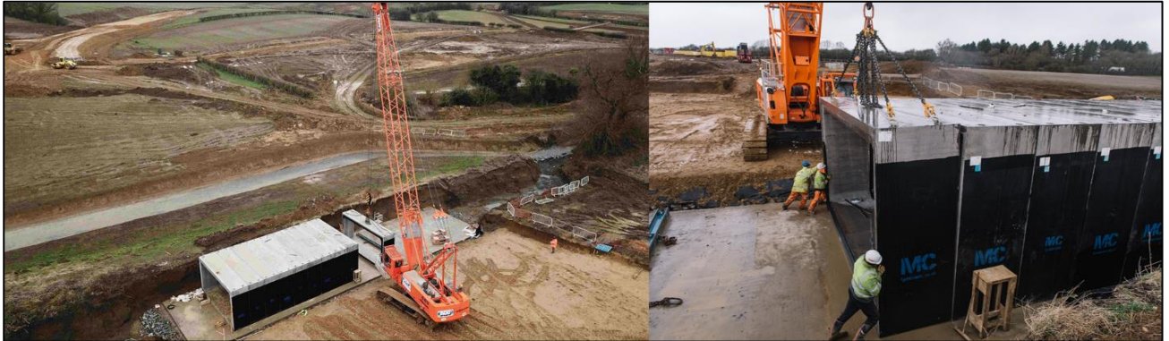
Diagram 2.4: Typical Box Culvert Construction – Sluice River Crossings
